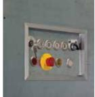
Recessed COP (Car Operating Panel) with hold-to-run push button, protected by a frame to prevent damage during loading operations.
